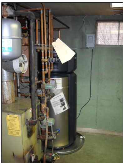
Figure 9. HPWH installed in boiler room
