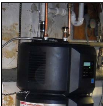
Figure 12. HPWH without heat traps
