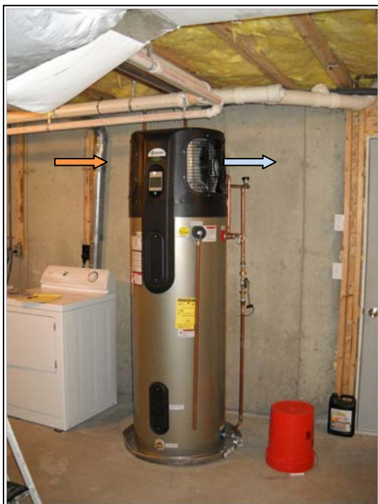
Figure 7. HPWH installed with adequate clearances
