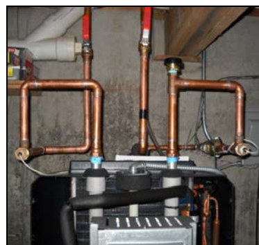
Figure 13. HPWH with heat traps
