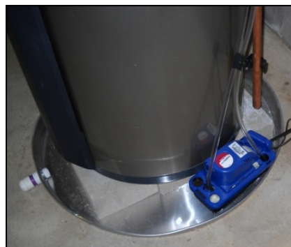
Figure 11. Proper HPWH installation
