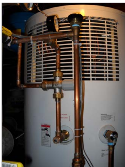
Figure 14. Heat pump water heater with mixing valve
