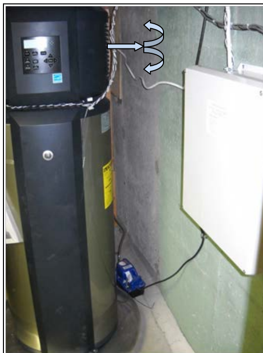
Figure 8. Improper HPWH with air discharge facing wall
