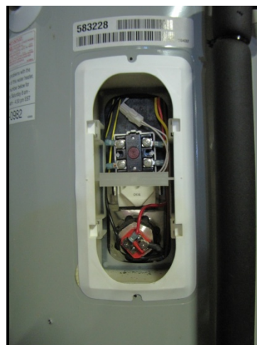
Figure 7. After the insulation is removed, the tank wall is accessible for installing a TC.
