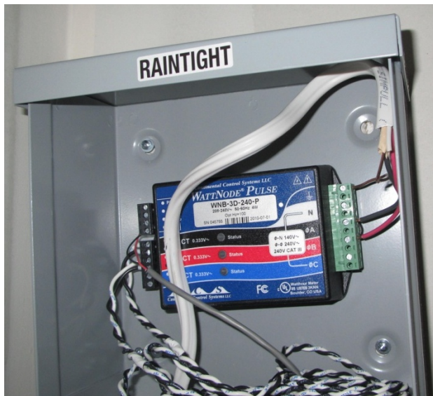
Figure 25. The wires from the CTs and the voltage tap are connected to the WattNode Watt-hour transducer.
